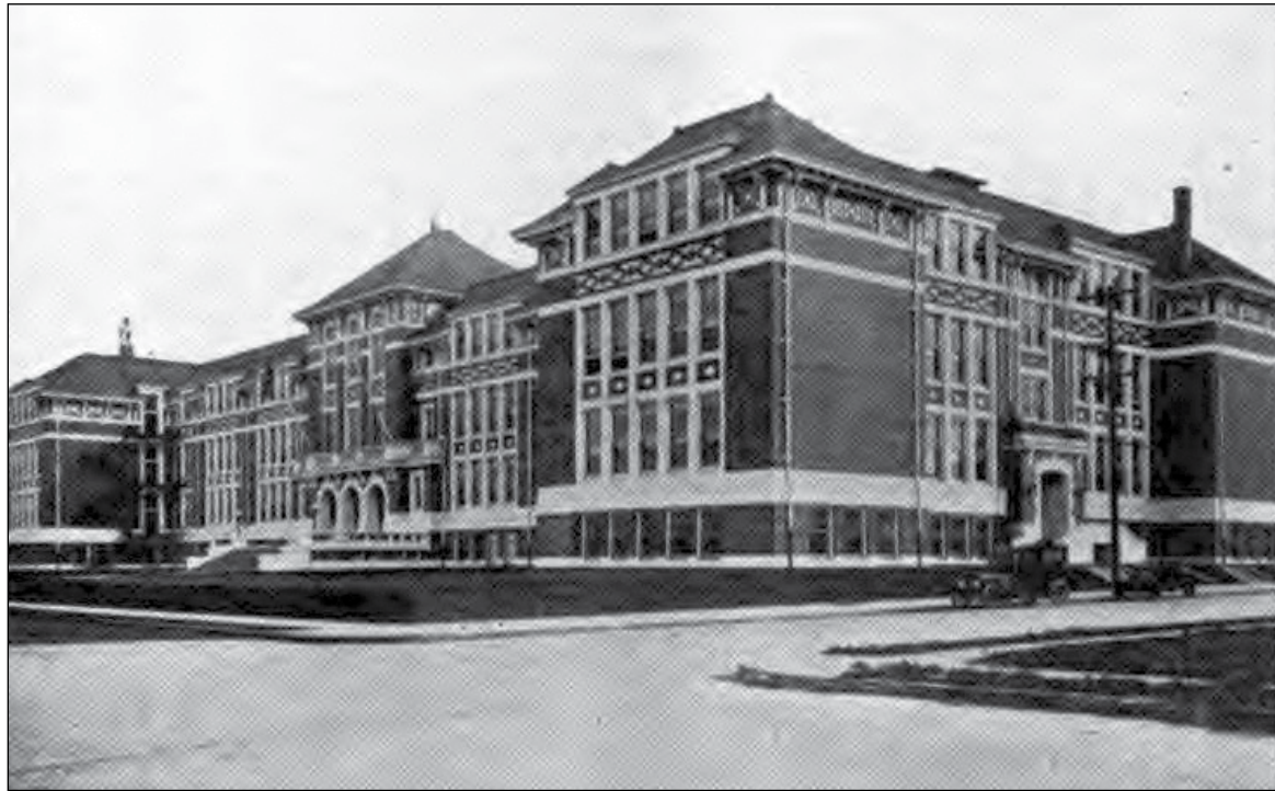
Jefferson High School was built in 1909. Engineers and architects determined that they couldn't reinforce the school's original four-story brick building safely and within the budget if students were inside. That prompted a plan to send students to Marshall High School while modernization work took place. Community members oppose the idea. (Wikipedia)
